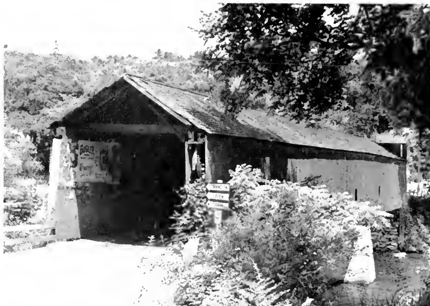
This covered bridge over the Housatonic links the towns of Sharon and Cornwall. It is one of the three remaining bridges of this type in Connecticut.
